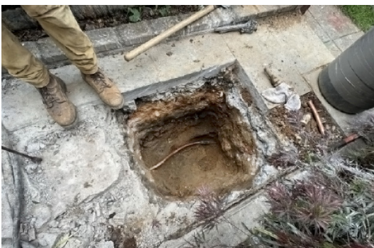
Test pit excavation at a residential property in DC
